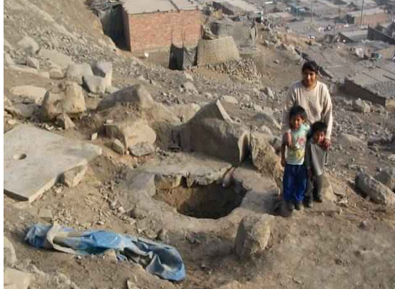
First you have to dig a 3 meter deep pit.
